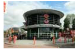
Walthamstow Bus Station
